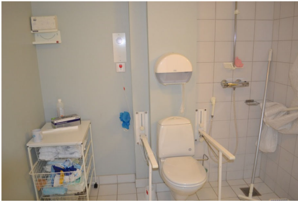
Fig. 3 A common location of toilet paper and flushing mechanisms. Picture from a nursing home built in 1997 (Boge 2014, page 62)
