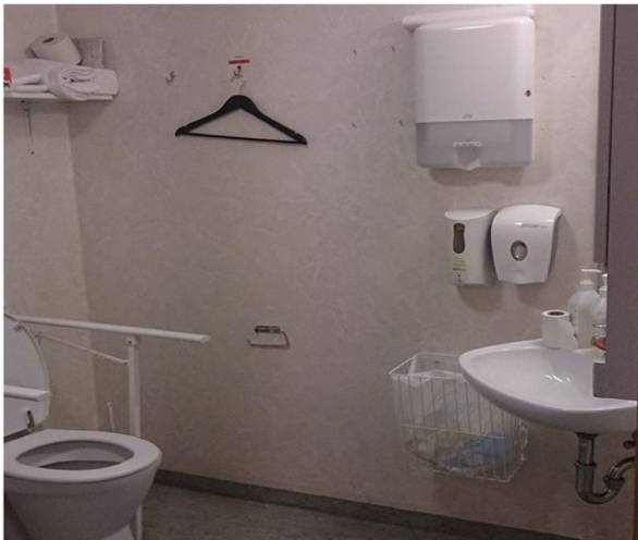
Fig. 6 A common placement of soap dispensers and paper towels. Picture from a nursing home that was built in 1992 (Boge 2014, page 78)
