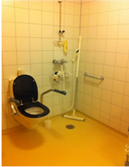
Fig. 1 A common toilet design. Picture from a Norwegian nursing home built in 2003 (Boge 2014, page 36)
